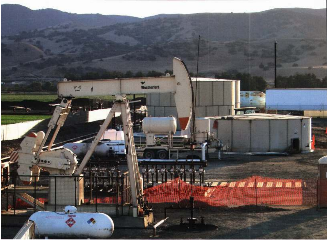
Salinas Energy's North San Ardo project
